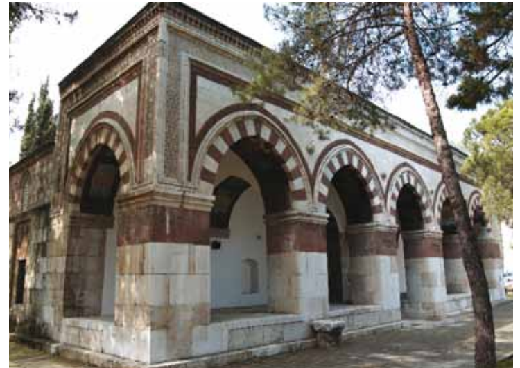
Bayezid Paşa Mosque
