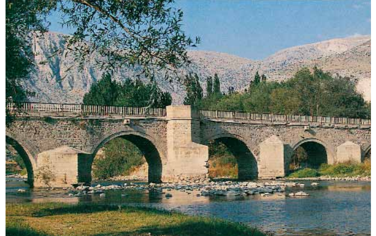
Çağlayan Köprü (Waterfall Bridge)
